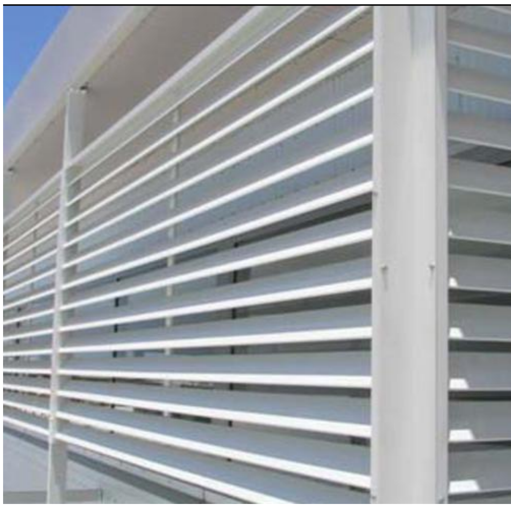
ROOF HVAC SCREEN
