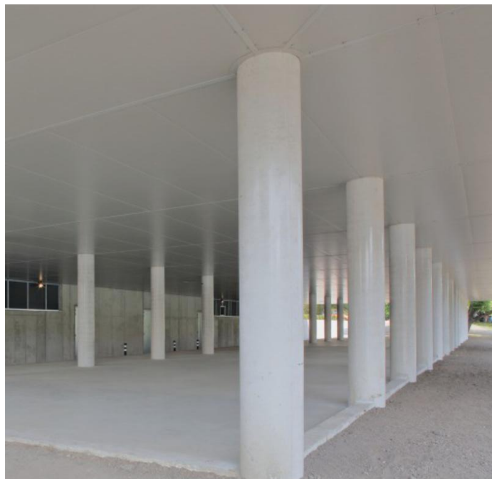
CONCRETE EXTERIOR COLUMNS
