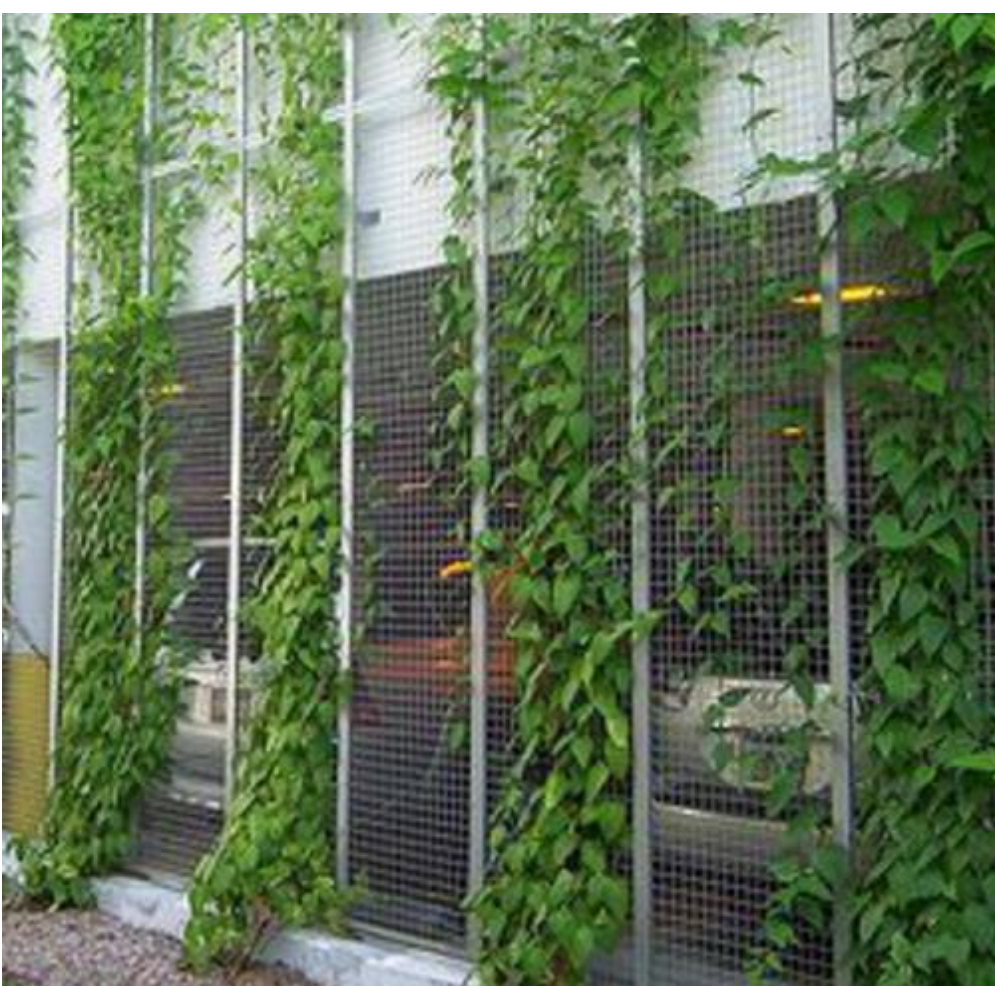
PARKING GARAGE GREEN WALL STUCTURAL SUPPORT
